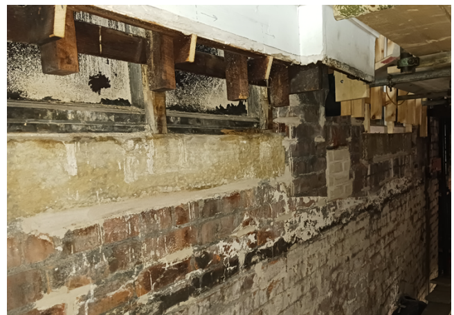
Removal of Cornice, Support Timbers and Wall Plaster
