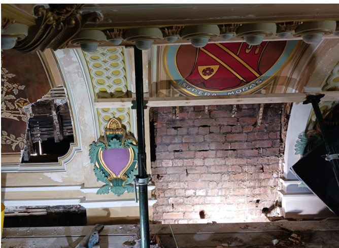
Partial Removal of Panels 1 and 2
